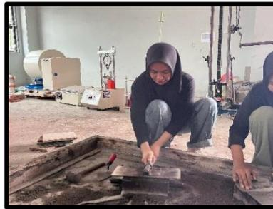
**Gambar 3.16** Pemasangan *paving block*
