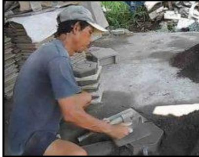
**Gambar 2.2** *Paving Block* Metode Manual (Asiacon, 2025)
